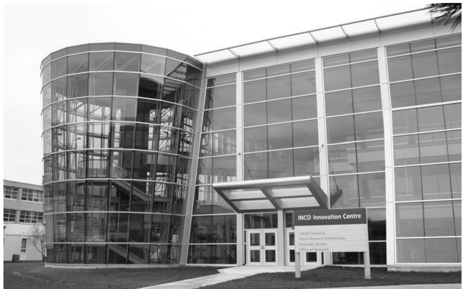
INCO Innovation Centre
